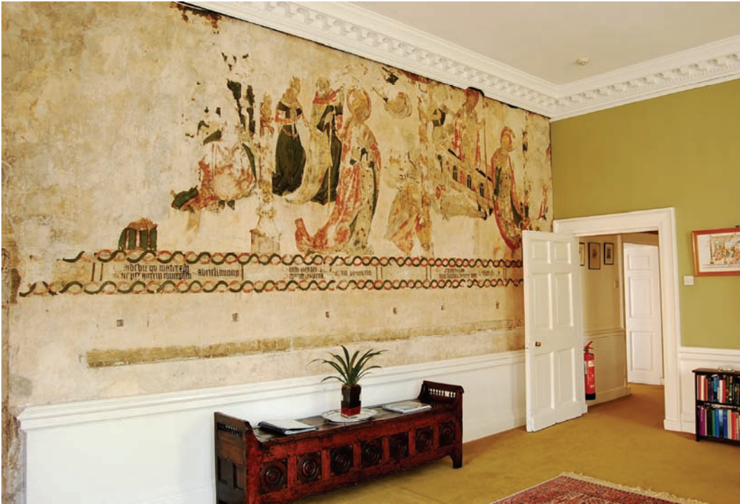
Fig. 4. The entrance Hall of the Deanery, the western end of the medieval Prior's Chapel.
